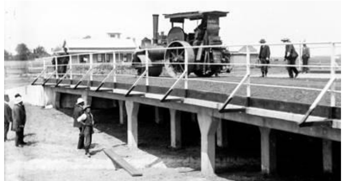
Reinforced Concrete T-girder Bridges. St Kilda Street Bridge, Elwood, Australia Load Test, 20 November 1905. University of Melbourne Archives GPNB/1094 Reinforced Concrete & Monier Pipe Construction Co Collection
