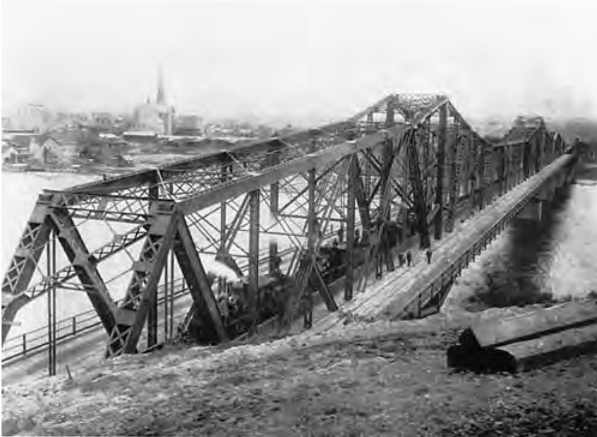
Interprovincial Bridge, Ottawa, Canada. View from Nepean Point looking towards Hull and showing the load testing of the bridge with four locomotives. This was the first run over the bridge on 12 December 1900. National Archives of Canada photo PA-202126.
